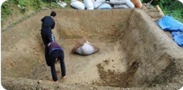
Figure 1. Smoothing of inner wall of Jalkund.
