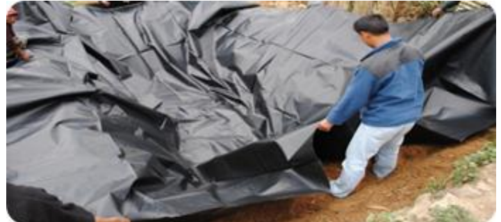
Figure 4. Laying of LDPE for Jalkund.
