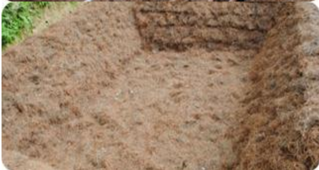
Figure 3. Cushioning of inner walls of Jalkund.
