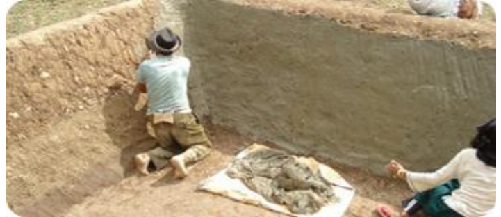
Figure 2. Plastering of inner walls of Jalkund.
