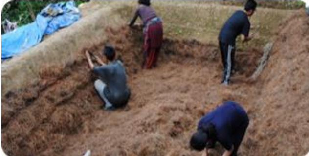
Figure 1. Smoothing of inner wall of Jalkund.
