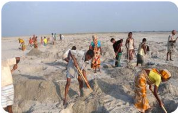
Preparation of Pit in Sandbar
